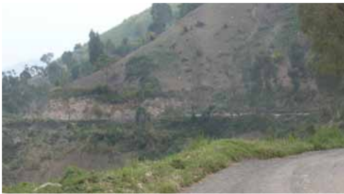
The road from Goma to Shasha, North Kivu, DRC. © Nadia Tabaro/WRC.
