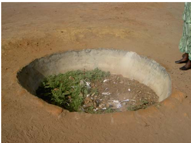
Unfenced medical waste pit, Health Centre II, Omot IDP camp.
