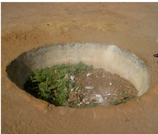
Unfenced medical waste pit, Health Center II, Omot IDP camp.
